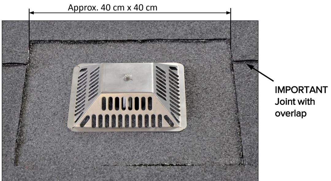
Figure 2 – Roof outlet fully installed with overlapping bitumen membrane lengths and leaf grate.
